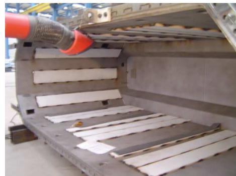
Assembled and painted (oil resistant special painting material) tank inside
