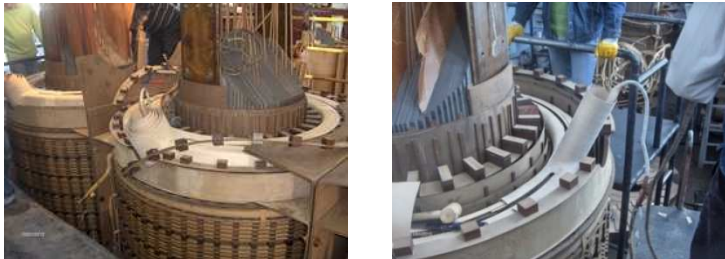
Figure15. Assambling of new upper end insulation parts
